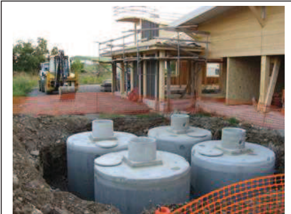
Figure 2. Concrete tanks (buried)
