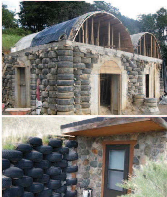
Illustration 2 Tyres being used to build a house
