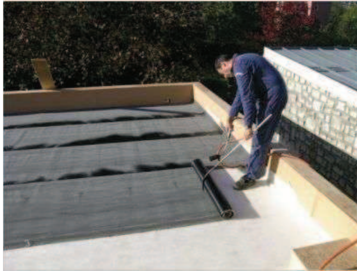
Illustration 1 Installation of waterproofing
