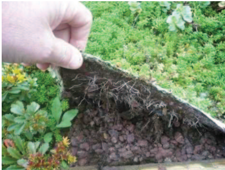
Illustration 2 A growing substrate and plant layer
