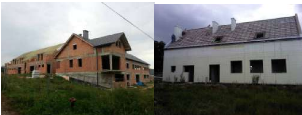
Community house in Rzeszow
