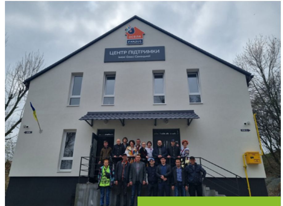
Emmaus Oselya's new social support centre and the whole team in February 2023. Construction work began in July 2022 and was completed in January 2023. Credit: Emmaus Oselya.
