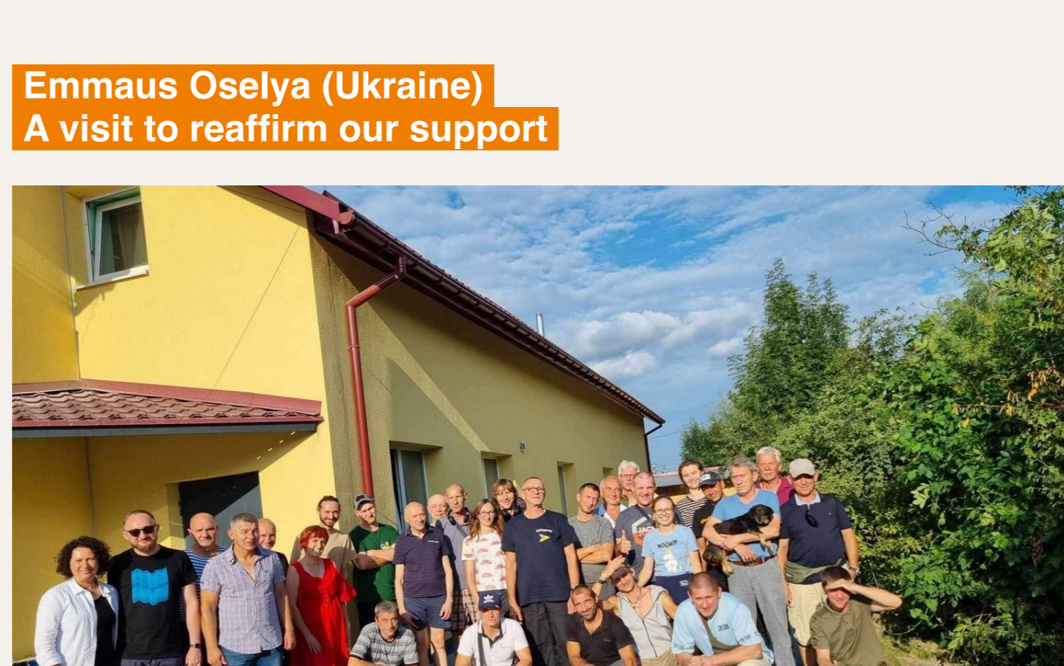
The Oselya community pictured in front of the community house extension, renovated in 2024 thanks to the Abbé Pierre Foundation and Emmaus Europe - Credit: Emmaus Oselya, July 2024.
