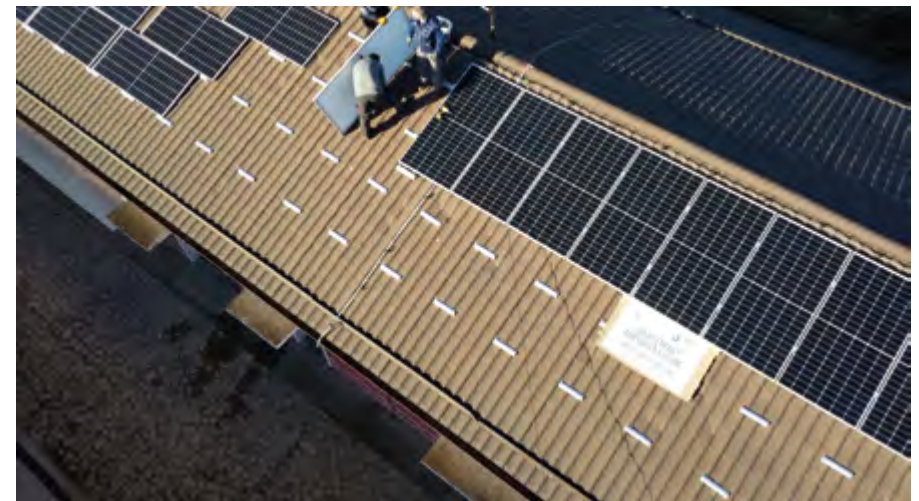
Emmaus-IFS Project – Solar Energy for a Green Future which led to the installation, in 2022, of solar panels generating over 25,000 kW of electricity per year.
